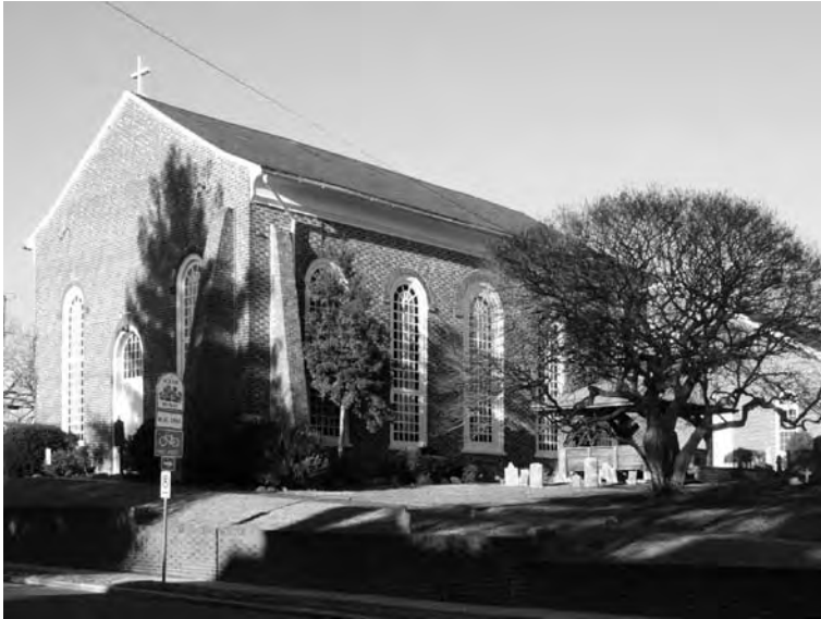
above: All Hallows Episcopal Church, built 1748-56 was initially funded by a 1748 levy of 80,000 pounds of tobacco, which raised approximately $1,064. The church, one of the most elaborate 18th century structures surviving on the Eastern Shore, required another levy of 45,000 pounds of tobacco to finish in 1756.
