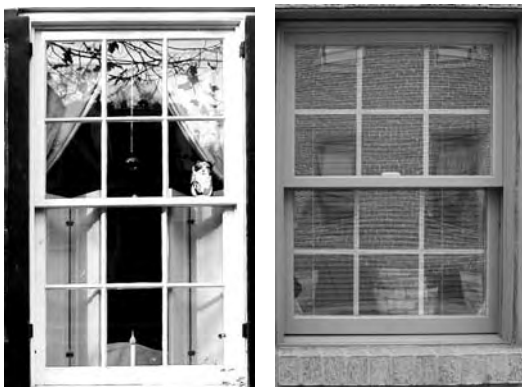
above left: Wooden window sash with individual panes of glass, held in place by muntins is the traditional and honest form of old-house window. above right: Plastic sash with fake muntins, often called "grilles" do not have the same character as the real thing.
