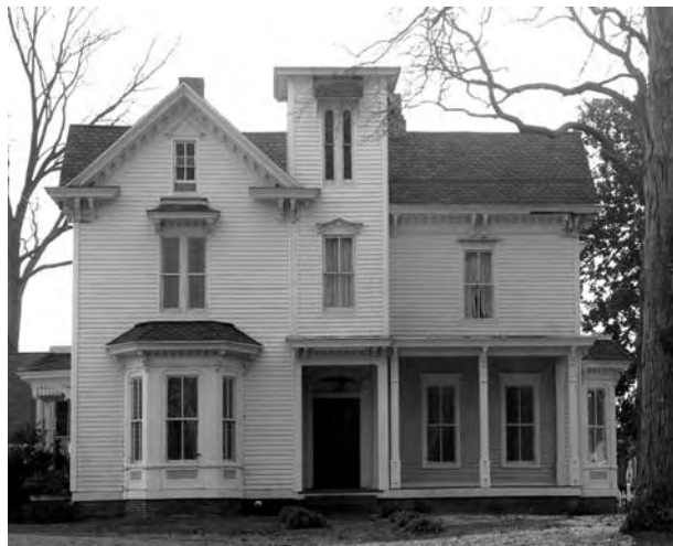
right: The George W. Covington house, built in 1878 is a relatively straightforward example of the Italianate style, and the façade with the tower in the center places it into the “Italian Villa” style. There was originally a roof on the tower, which would add much to the look of the house if it were to be restored. Replacing an important missing part of a historic building, using old photographs and evidence from the period is what is properly referred to as a restoration as opposed to a repair or renovation and should be undertaken carefully with advice and approval from the HDC.
