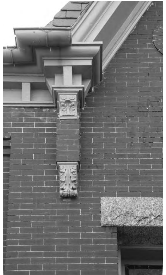
Decorative cornice details and brackets
