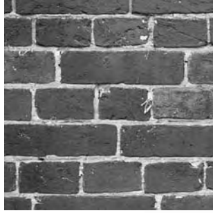
18th - early 19th C. soft brick English bond, rake pointing
