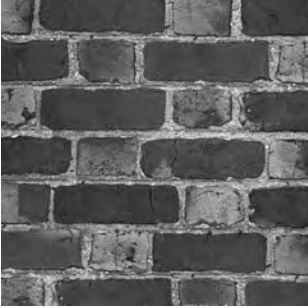
18th C. brick, Flemish bond glazed headers All Hallows Episcopal Church photo Karen Houtman
