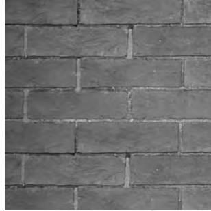
19th C. soft brick common bond, red mortar Mackemie Presbyterian Church photo Karen Houtman
