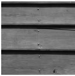
above: 18th century beaded clapboard with handmade nails
