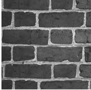
18th C. brick, Flemish bond unglazed headers All Hallows Episcopal Church photo Karen Houtman
