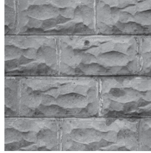
Home-made concrete block, made with a Sears Roebuck mold, an endangered material. Purnell Shockley house
