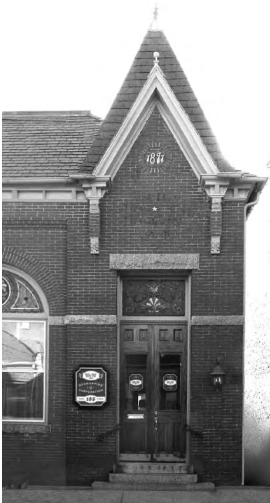
above: An unusual commercial building (1897) with a steep pitched turret above the oak doors. The building is constructed of rubbed brick with narrow mortar joints and granite belt courses and steps.
