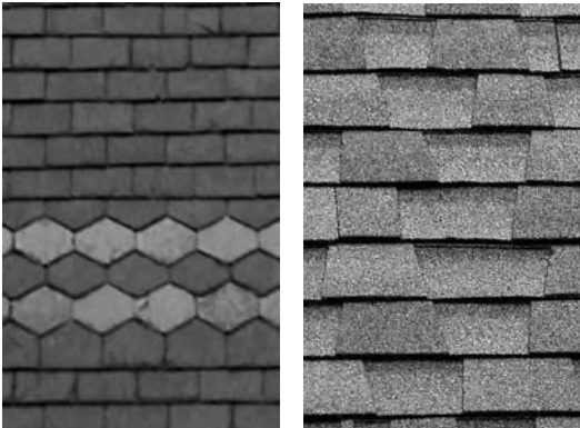
above left: Slate is a natural material. A slate roof can last hundreds of years. above right: Asphalt "architectural" shingles look nothing like slates in texture or scale and are a poor substitution.
