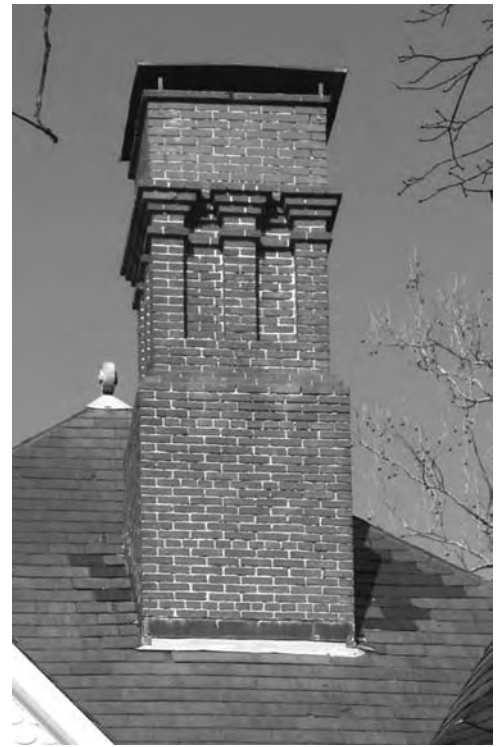
right: Corbeled chimney stack on the Governor John Walter Smith House, 1890. Chimneys such as these were a defining feature of the Queen Anne style in America.
