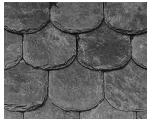
above: Slate is a natural material. A slate roof can last hundreds of years.
