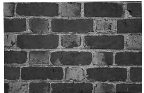
above: Glazed headers in Flemish bond. All Hallows Episcopal Church. photo Karen Houtman
