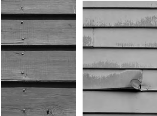
above, left: Wooden siding is a traditional building element and an honest material. above right: Aluminum or vinyl siding is a poor imitation, eventually needs to be painted, and cannot be repaired when cracked or dented.
