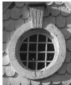
Original wooden windows and trim
