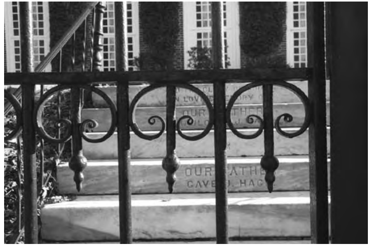
Original wrought iron fence and gate
