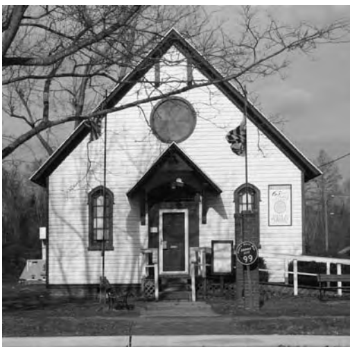
below: Built in 1891 as a Catholic Church, this building now houses the Julia A. Purnell Museum, a remarkable collection of needlepoint and other historic artifacts. The interior is an unusual open scissor-truss structure with iron tie rods.
