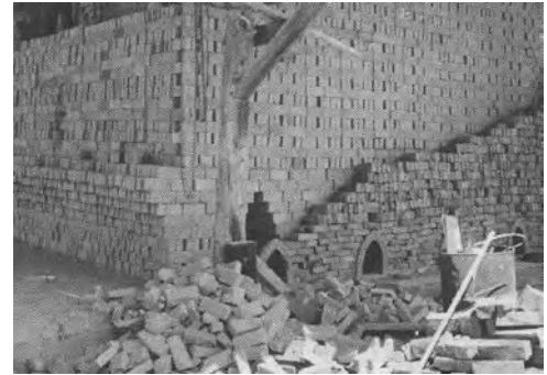
above: Scove kiln for firing bricks. photo Philip Marshall; Masonry the Preservation Press
