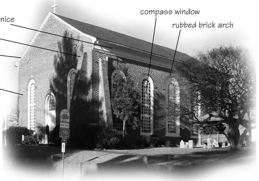
above: All Hallows Episcopal Church, 1748-56 one of the high style surviving mid-18th century churches on the Lower Eastern Shore, the building is built in the most elaborate style of the period, Flemish bond with glazed headers, giving a checkerboard effect.
