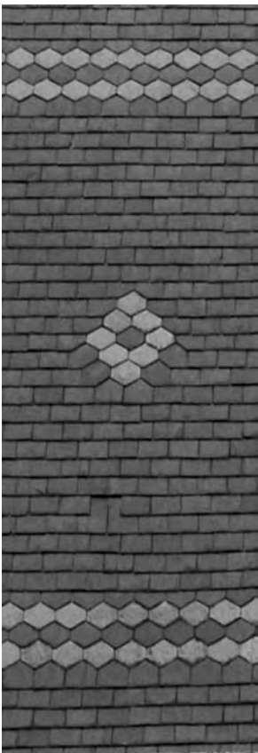
Decorative slate roofs
