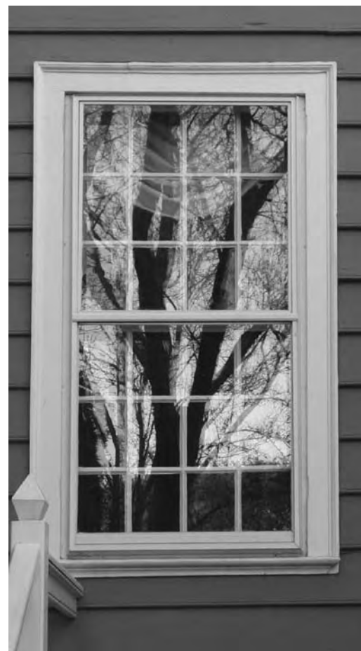
above: Historic wood windows, with sound putty, reasonable weatherstripping and exterior storm windows have the same energy efficiency as vinyl thermal-pane windows.
