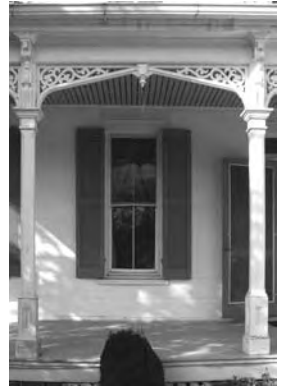
above: Typical Gothic revival porch trim; chamfered posts, Tudor style 4-centered arch with tracery and spindles
